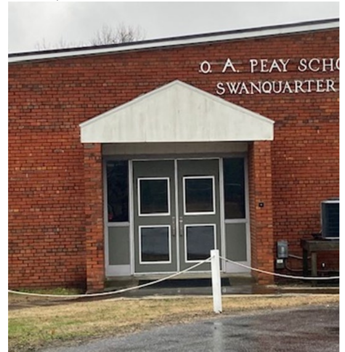
Roof C, photo #11
