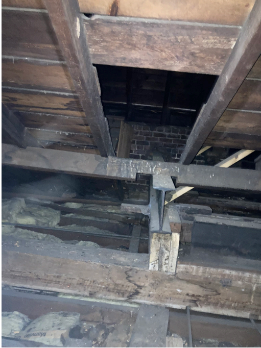
Dormer Attic Interior Access
