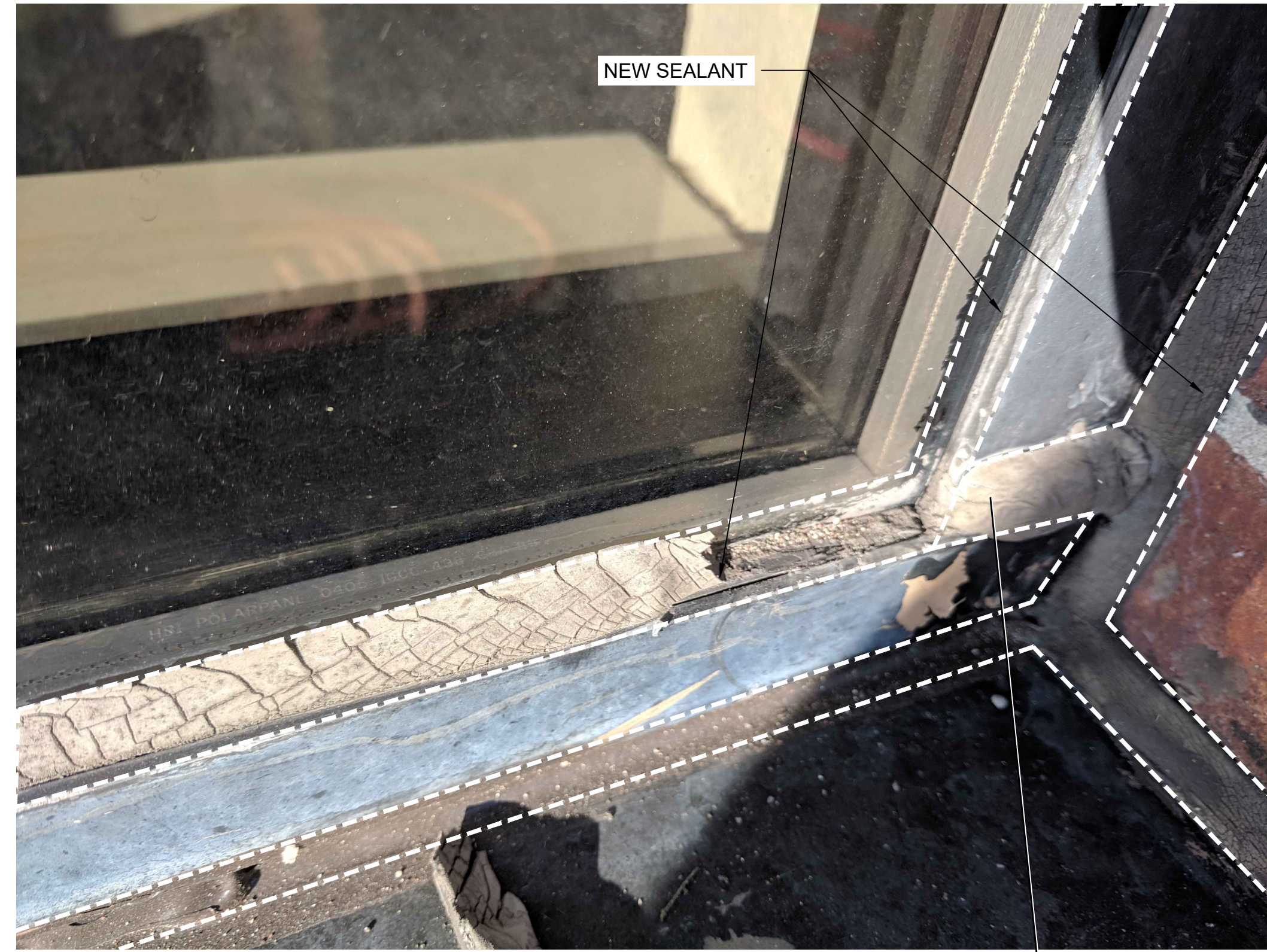
2 WINDOW SEALANT DETAIL Scale: NTS
