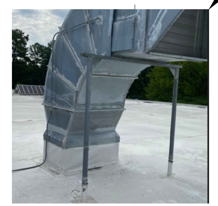
CONDITION OF DUCT PENETRATION 2.1
