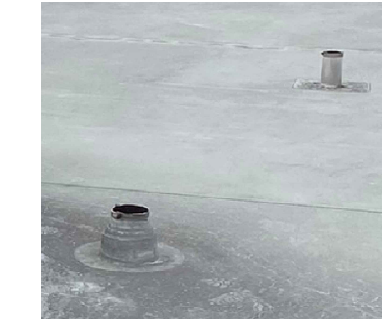
TYPICAL ROOF VENT CONDITION
