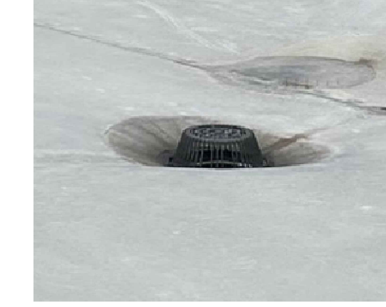
TYPICAL ROOF DRAIN CONDITION
