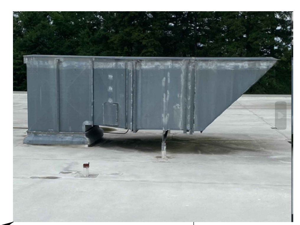
CONDITION OF DUCT PENETRATION 2.4
