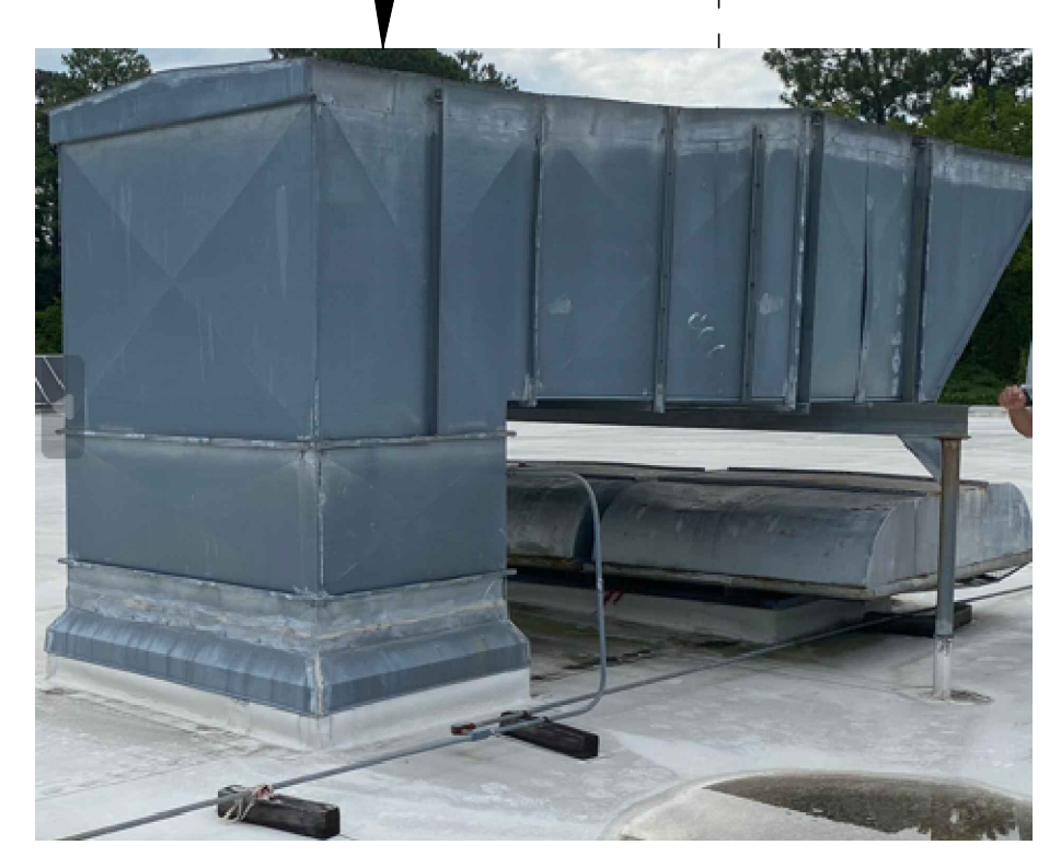
CONDITION OF DUCT PENETRATIONS 2.2 AND 2.3
