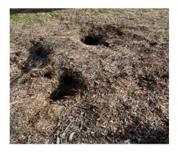
Contractor to remove in its entirety, add acceptable fill dirt, grade to provide positive drainage and install Bermuda sod with 4-inches (min.) topsoil. This work is to be included as part of the base bid. (item #27F from Addenda)
