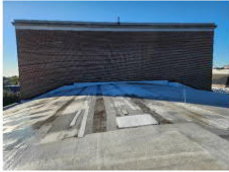
Photo #1 Barrel Roof and High Building on south side (Roof 1)
