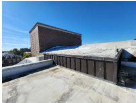
Photo #4 Upper and Lower Flat Roofs on NE side (Roofs 2 and 4)
