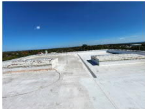
Photo #6 High Building Roof (Roof 7)
