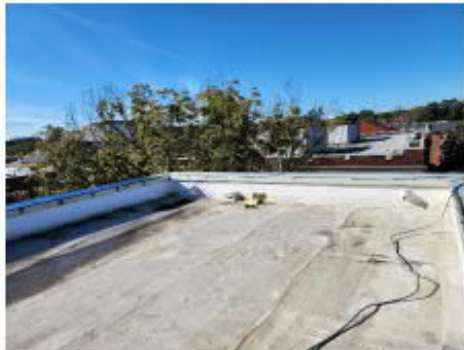
Photo #3 Lower NW Flat Roof (Roof 3)
