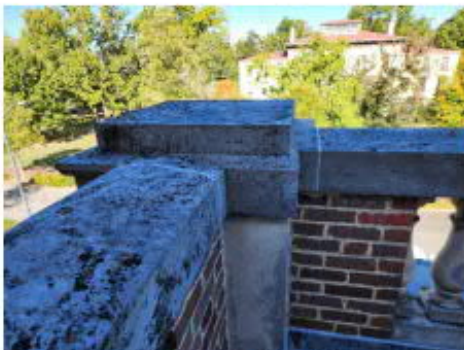
Photo #11 Asbestos-containing White Caulk on Balustrade at the North Porte-Cochere Roof 9 (HA #21)
