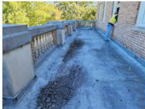
Photo #5 North Porte-Cochere Roof with Balustrade (Roof 9)
