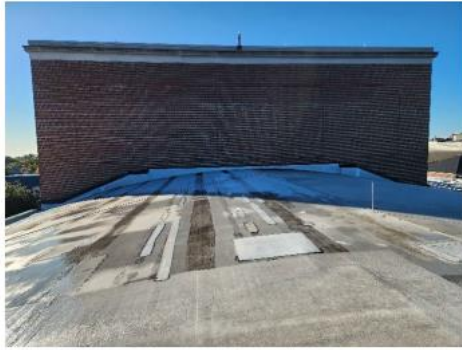
Photo #1 Barrel Roof and High Building on south side (Area A)
