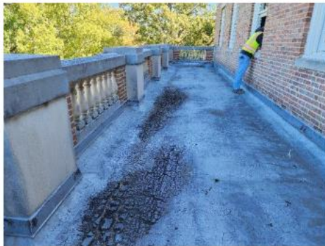
Photo #5 North Porte-Cochere Roof with Balustrade (Area 9)
