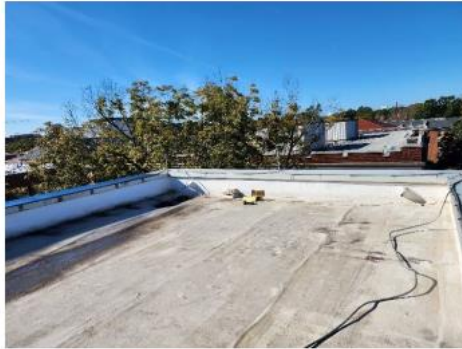
Photo #3 Lower NW Flat Roof (Roof Area 3)
