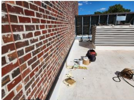
Photo #7 S-SE Low Roof with Metal Screen Wall (Area 8)
