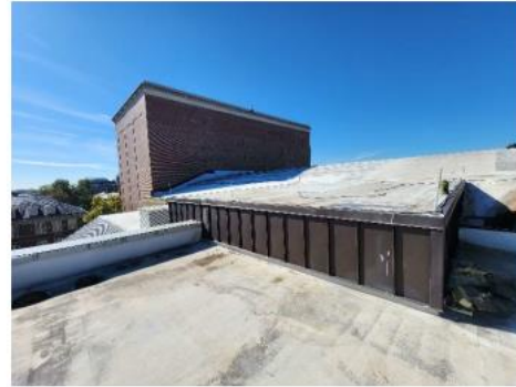
Photo #4 Upper and Lower Flat Roofs on NE side (Areas 2 and 4)
