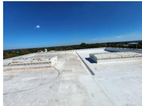
Photo #6 High Building Roof (Area 7)
