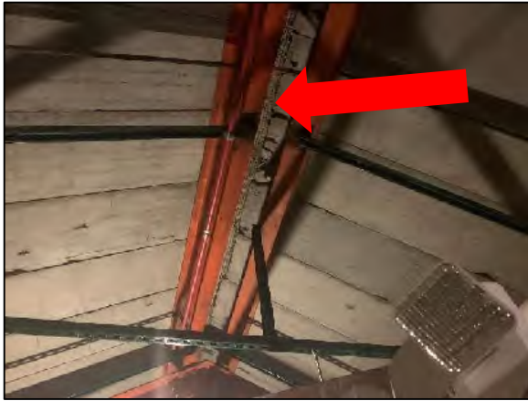
General location of asbestos containing seam grout filler (typical).
