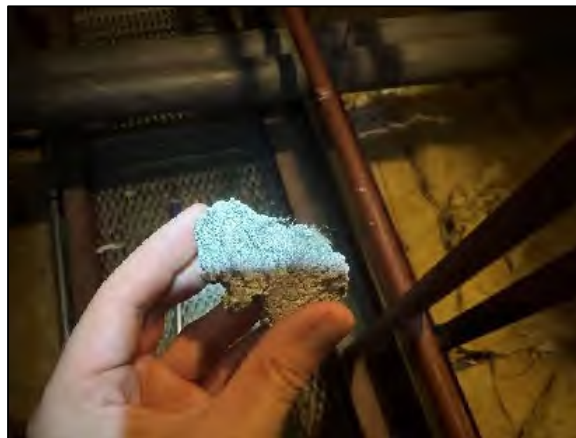
PHOTO 2 Close-up view of Sample BB-1 Central Wing - Attic 2% Chrysotile
