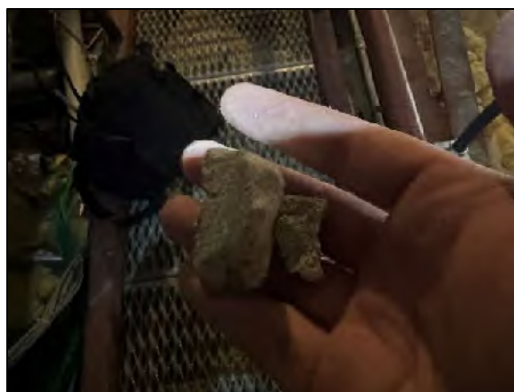
PHOTO 4 Close-up view of Sample BB-2 Central Wing - Attic 2% Chrysotile
