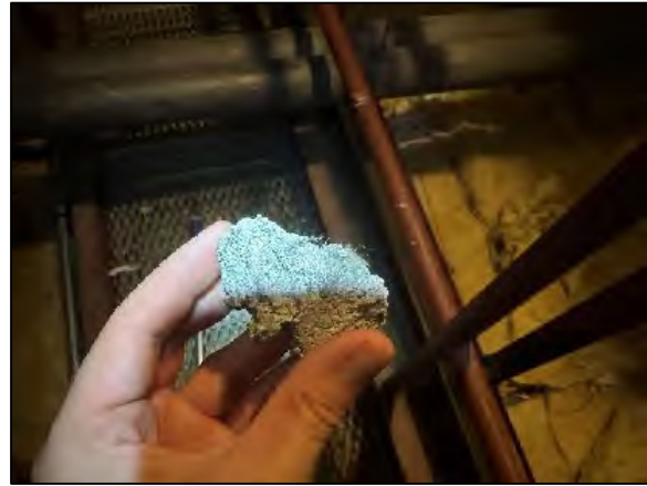
Close-up view of asbestos containing seam grout filler (typical).
